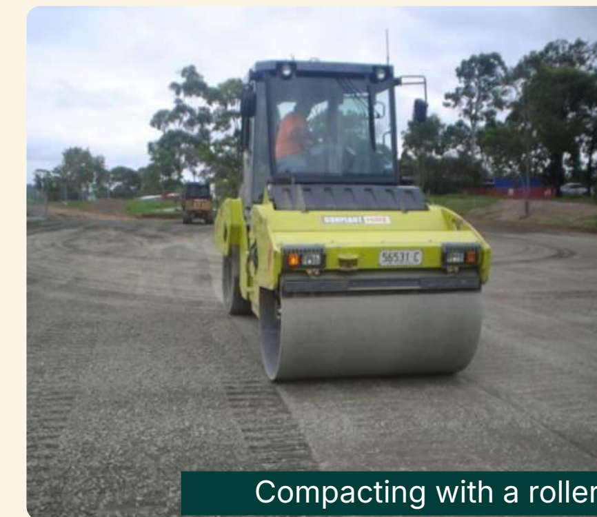
Importing the crushed rock layers – sub-base
