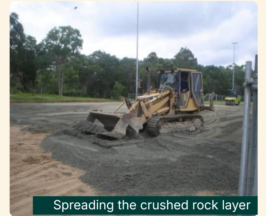
Importing the crushed rock layers – sub-base
