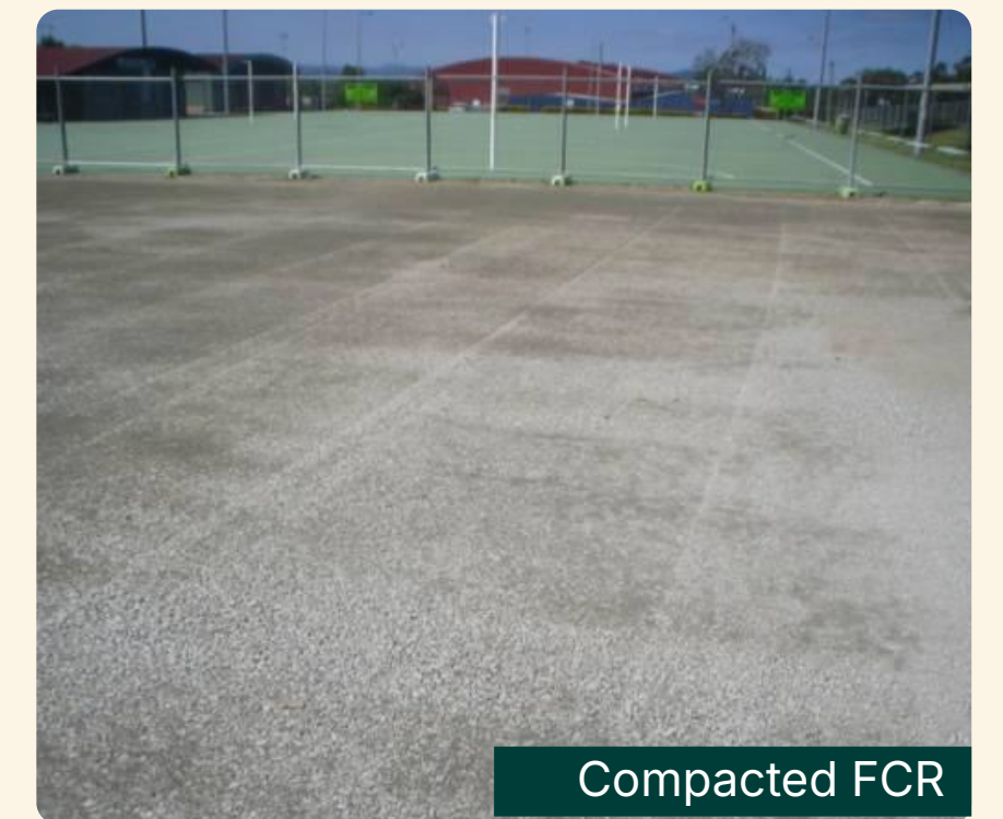
Compacting with a roller
